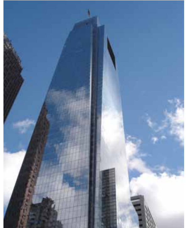
2.1 million feet of cabling and 27,000 AMP-TWIST jacks are installed in the Comcast Center.
